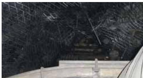
Manifestations of rock pressure in the mining entries: а – deformations in the form of roof sagging in the excavations supported by single-level roof bolts; б – roof doming in the excavations with combined support
